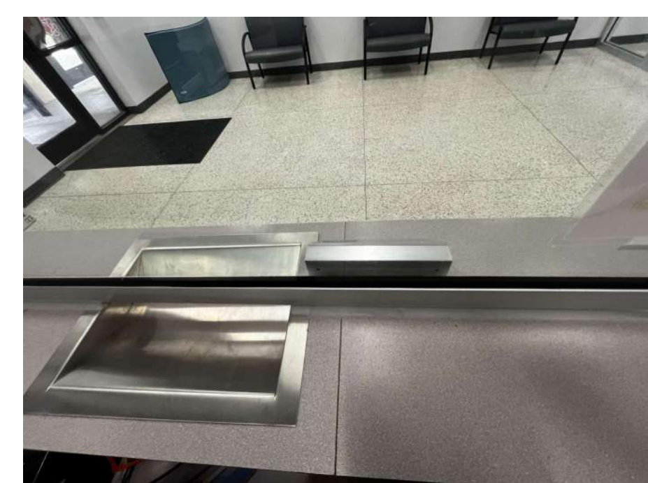
IMG_8279 SALVAGE 2 RECEPTION AREA COMMUNICATION BOXES
