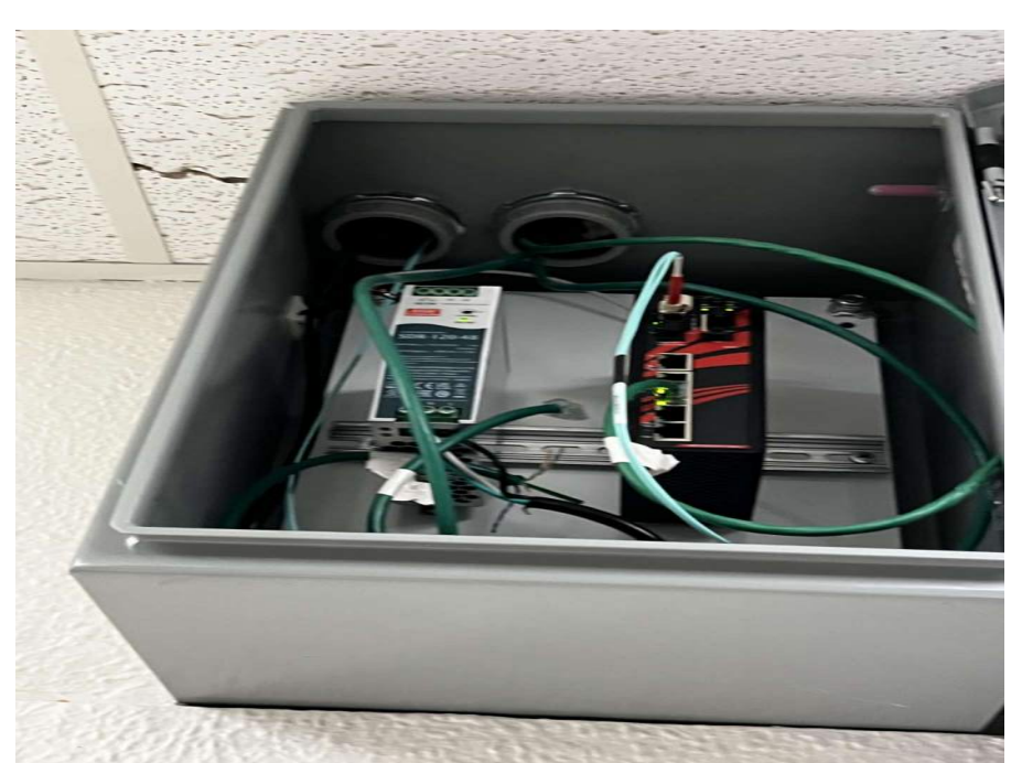
IMG_8264 SALVAGE INTERNALS AND BOX
