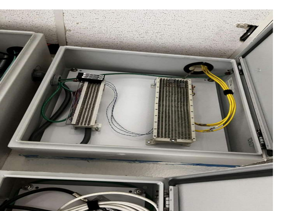
IMG_8262 DEMO INTERNAL SALVAGE BOX
