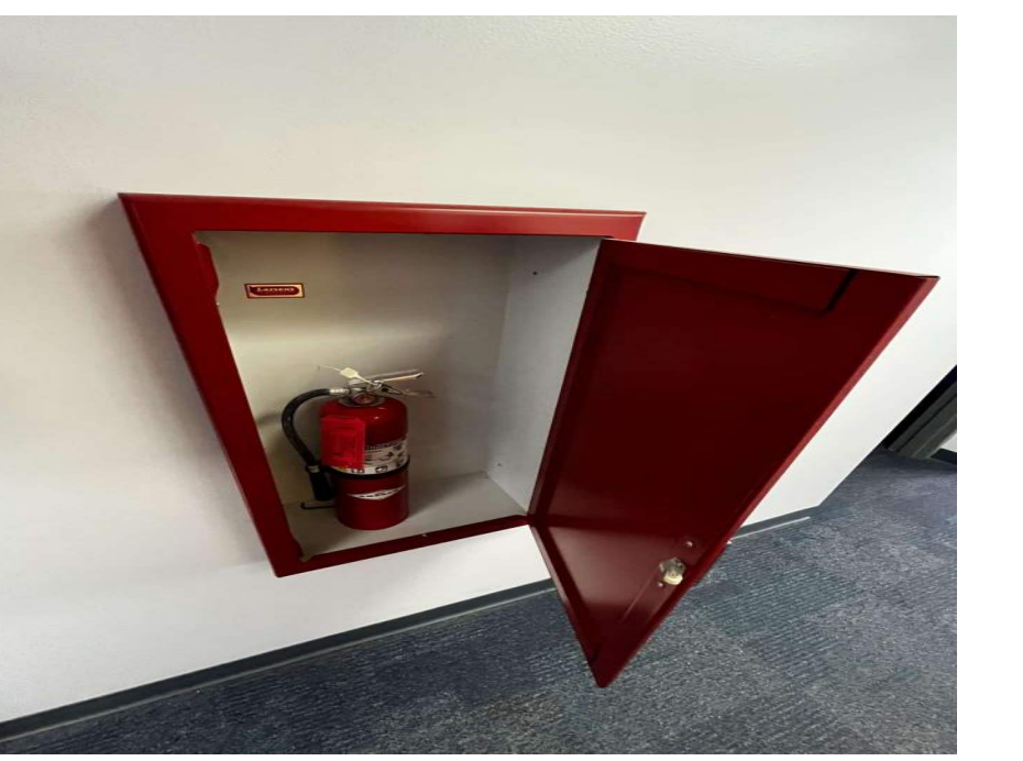
IMG_8283 SALVAGE ALL FIRE EXTINGUISHERS DEMO CABINETS
